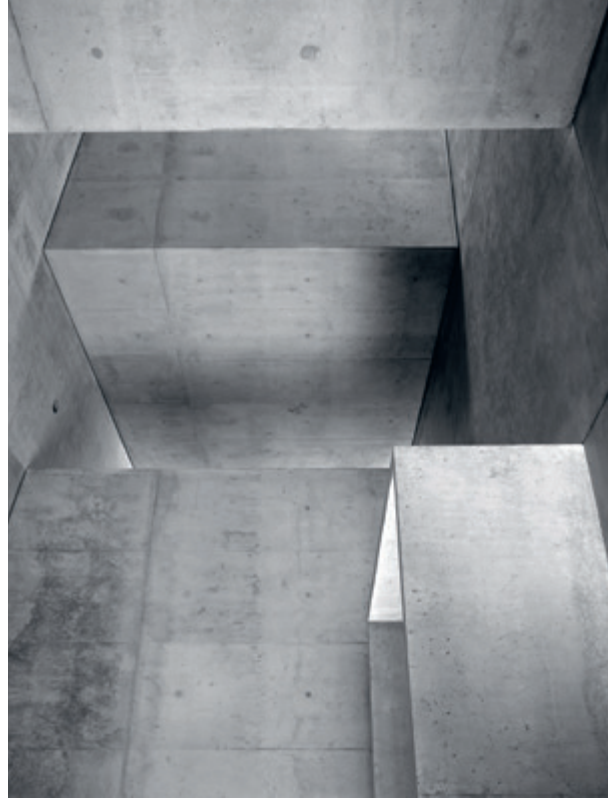
PROJECT: SCHOOL ARCHITECT: VALERIO OLGIATI LOCATION & YEAR: PASFELS (GR), 1996–1998 IMAGE: HEINRICH HELFENSTEIN © 2016, PROLITTERIS, ZÜRICH
