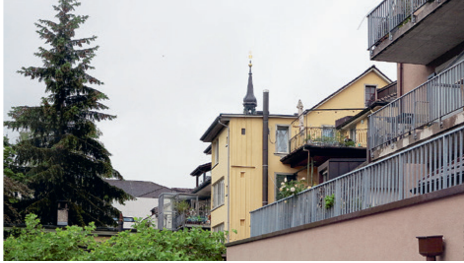
PROJECT: REAR SIDE OF THE HISTORICAL CENTRE OF FRAUENFELD LOCATION: FRAUENFELD (TG) IMAGE: PHILIPP BOLLIER, AGPS ARCHITECTURE (3)
